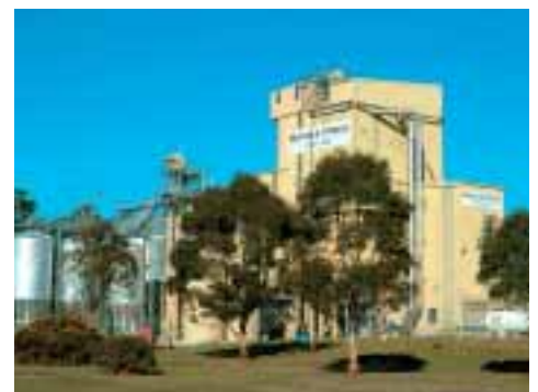
Monds and Affleck Processing Plant, Westbury
