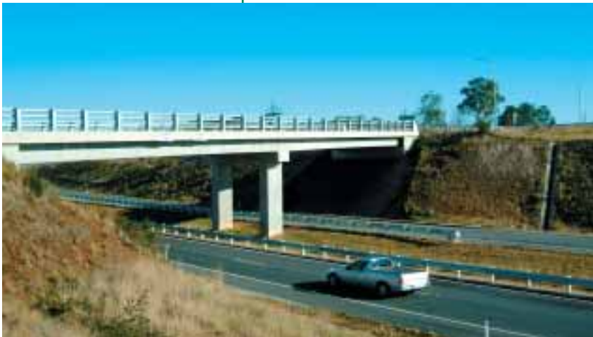
Westbury Bypass, Bass Highway
